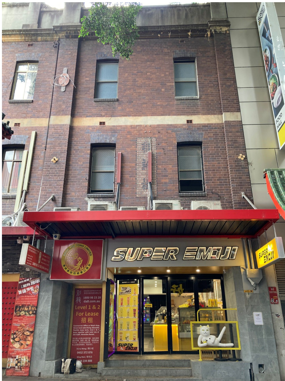
Figure 30. View of 54 Dixon Street. Source: HAA, 2024.
