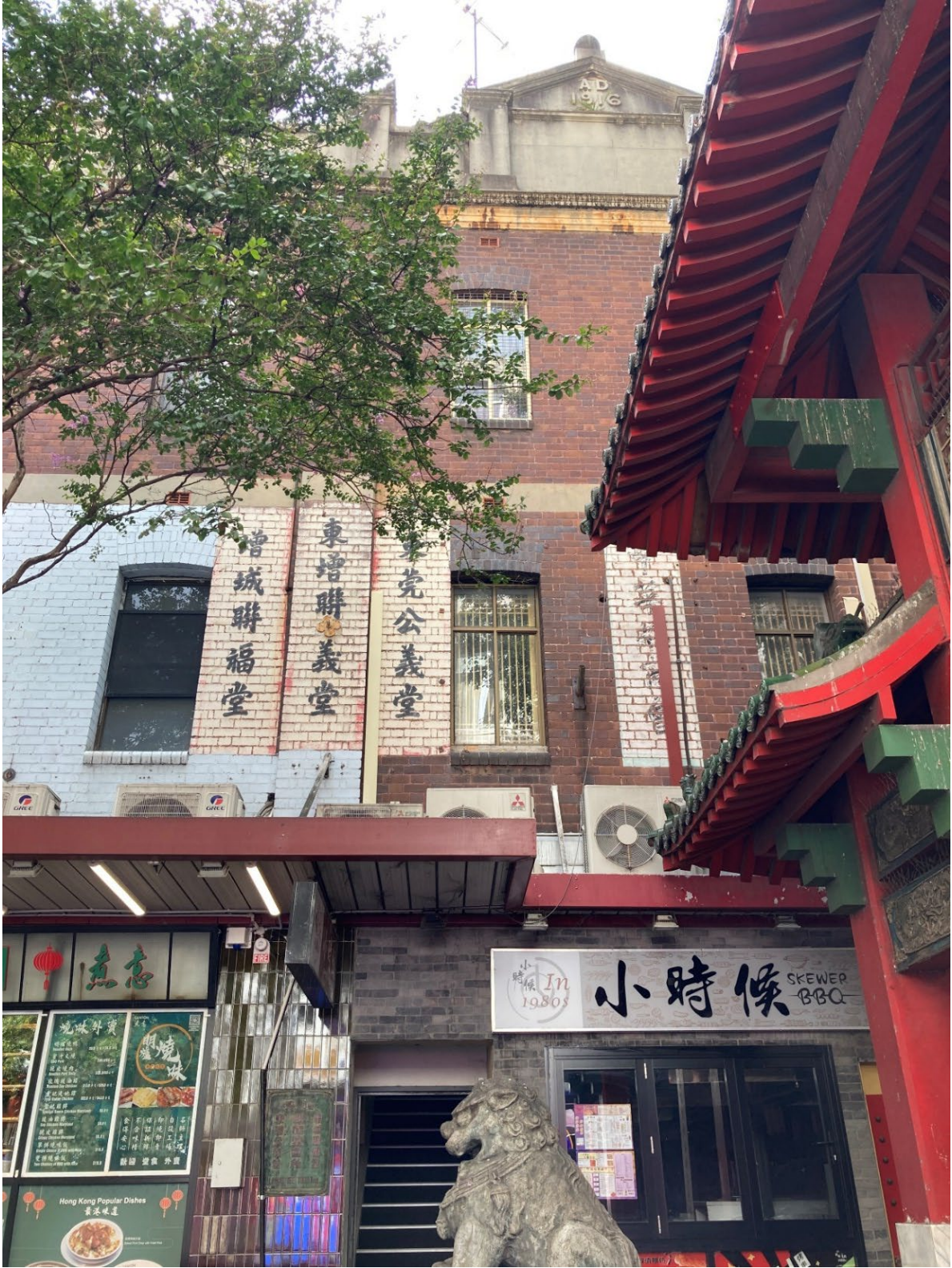
Figure 28. View of 52 Dixon Street. Source: HAA, 2024.
