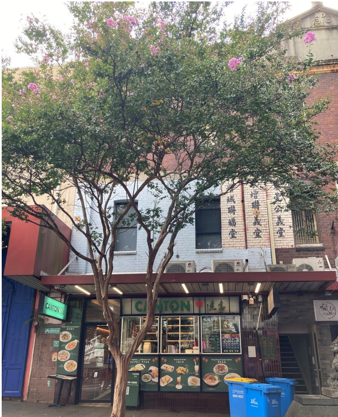
Figure 26. View of 50 Dixon Street. Source: HAA, 2024.
